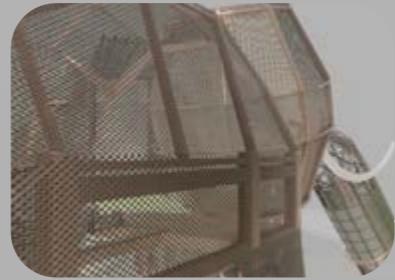
Steel frame covered with metal mesh
